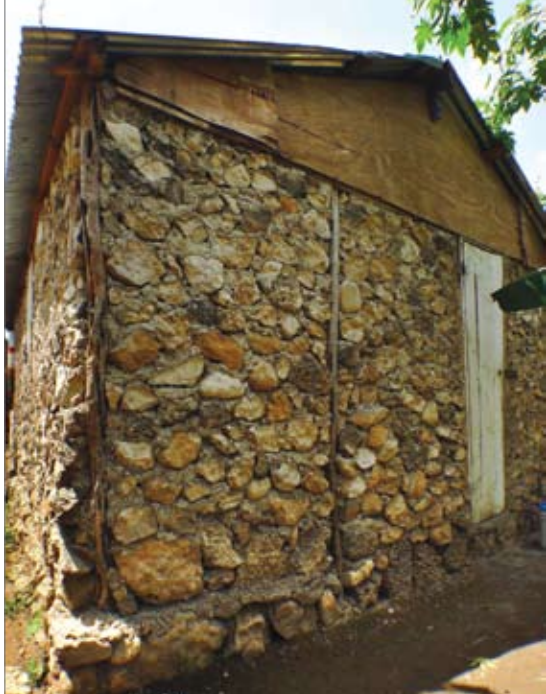
Timber frame house with stone-and-mortar infill.
