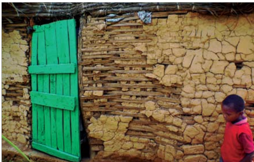
Wattle-and-daub house. Building in the vernacular style may be one way to help communities feel validated and have access to development now.
